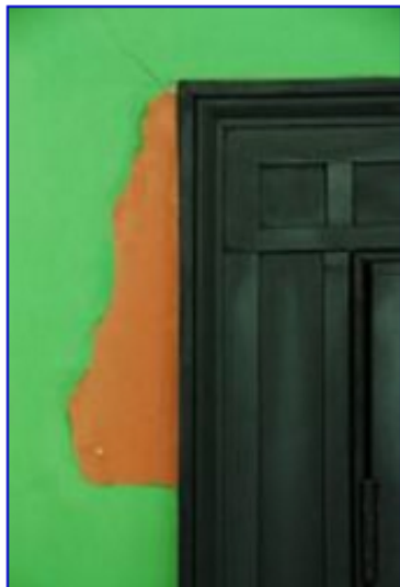
Weir Farm Closet Before (contributed photo)
