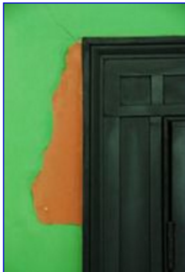
Weir Farm Closet Before (contributed photo)
