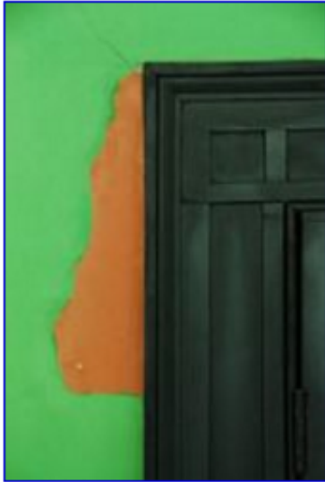
Weir Farm Closet Before (contributed photo)
