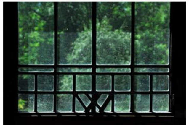
Design and placement of traditional lead-cane stained-glass windows served to unite the Weir House with the landscape. (Photo © 2011 www.xiomaro.com)
