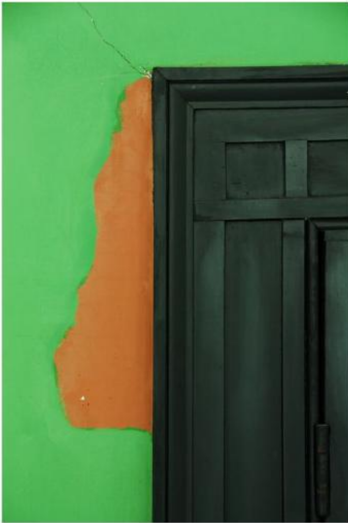
Closet door before restoration
