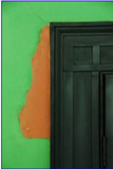
Weir Farm Closet Before (contributed photo)
